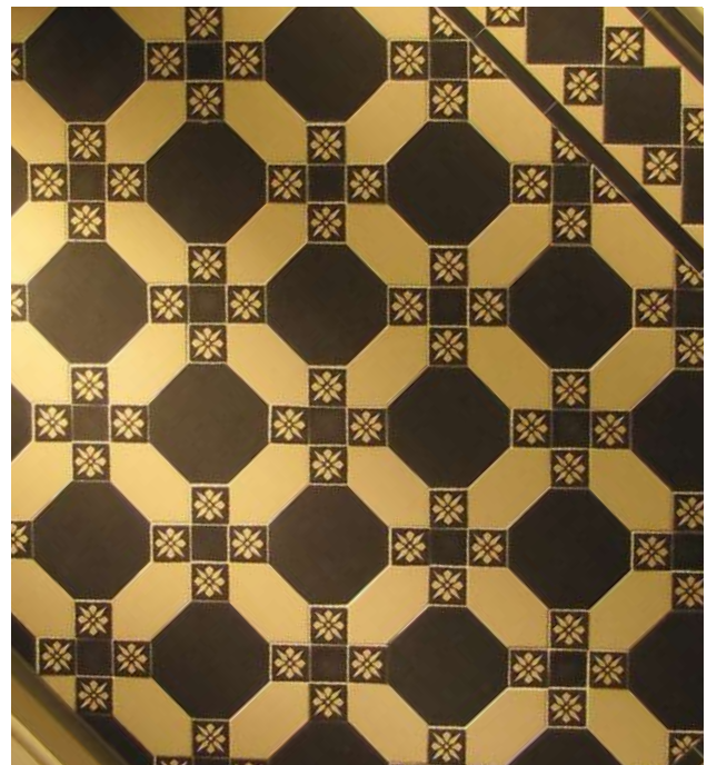
v Below: use of encaustic tiles within assemblies (borders and floor designs).
