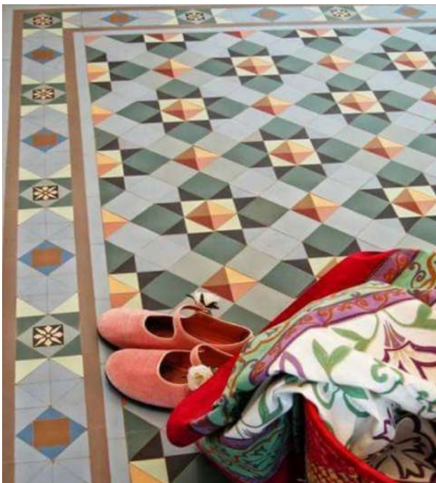
v Below: use of encaustic tiles within assemblies (borders and floor designs).
